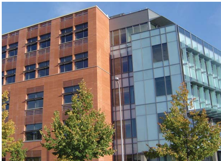
Southwest corner viewed from Boat St.
